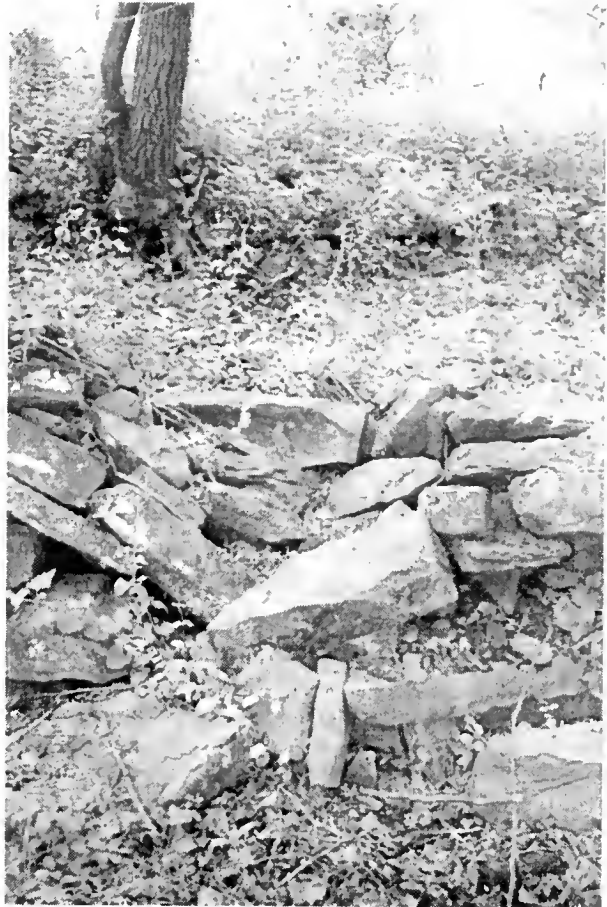
Figure 47 Stonework of the Dam, 2001
